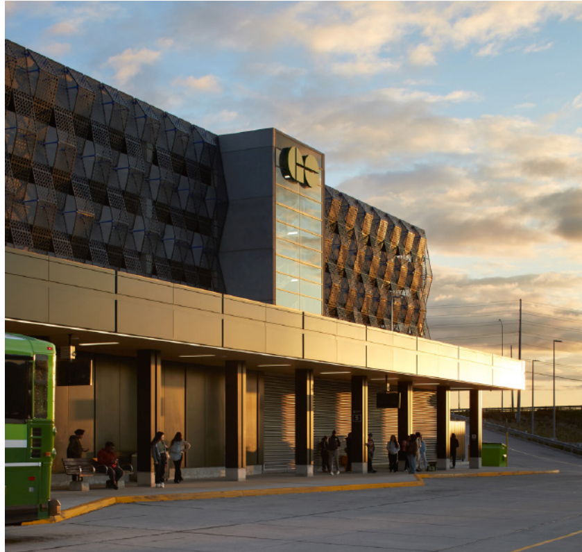
Bramalea GO Station Parking Building, Brampton, Ontario 2024 Award of Excellence Winner Apex Award, Architectural Design
